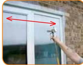
**4.** Release the trigger at the end of each stroke. Then depress the trigger and overlap the previous pass by 50%. Continue in this fashion for consistent coverage working down the substrate.
