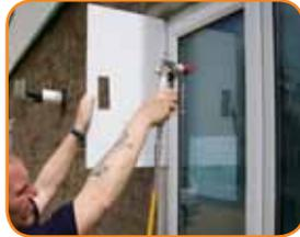
**3.** Release the safety catch and start spraying in a horizontal direction. Keep the gun at right angles to the surface. This means moving your entire arm back and forth rather than flexing the wrist.
