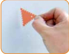
**6.** Use a wet film gauge to check that the coating's wet film thickness (WFT) is at least 10 Mils. Remove any masking tape while the product is still wet.
