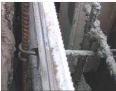
Stay-Form blind side wall tie using RH-6's and LC-6 Loop-Coil Ties.
