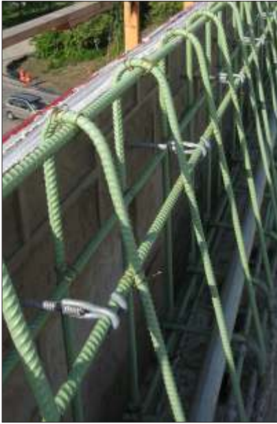
Attachment of plywood-backed form liners for slip-formed highway barriers. Galvanized RH-6.
