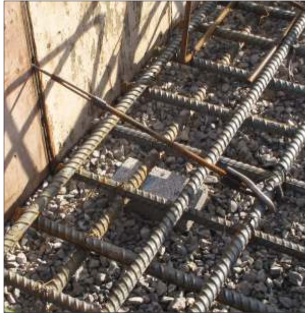
RH-48 Rebar Hooks and LCT-7 Turnbuckle ties used to tie Steel Ply edge forms to rebar mat on 20' x 30' x 3' slab pour.
