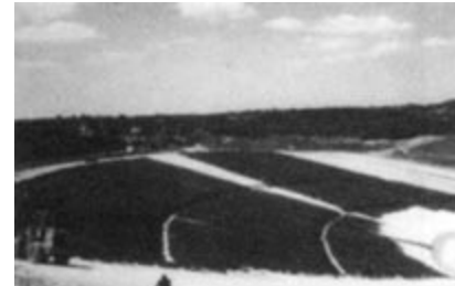
Mirafi® N-Series heavyweight nonwoven used as a liner protection in landfill application
