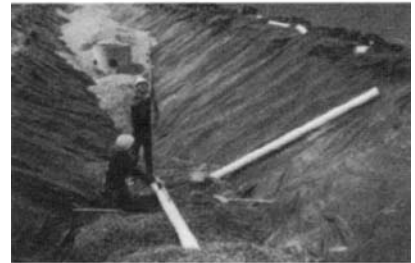
Mirafi® N-Series light weight nonwoven used as protective filter in an athletic field
